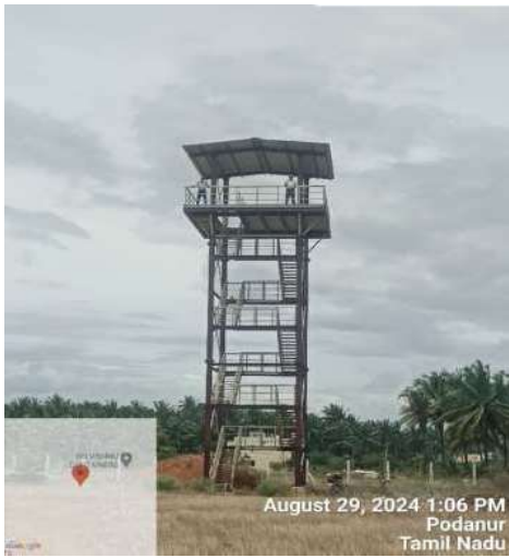
Watch Tower in Vellalore Compost Yard
