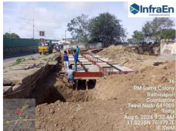
preparing the reinforcement for ramp construction - Sathy road transfer station
