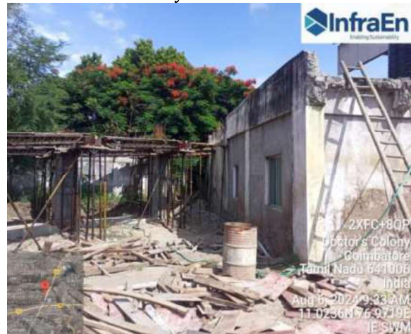
Lintel reinforcement work going on - Sathy road transfer station
