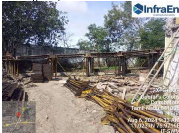
Lintel reinforcement work going on - Sathy road transfer station
