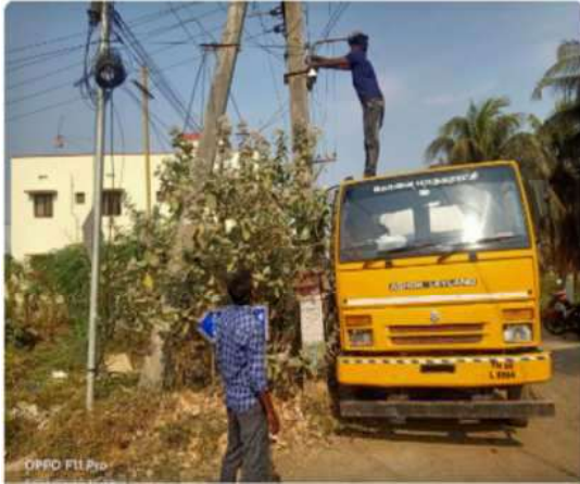
CCTV Installation & Surveillance
