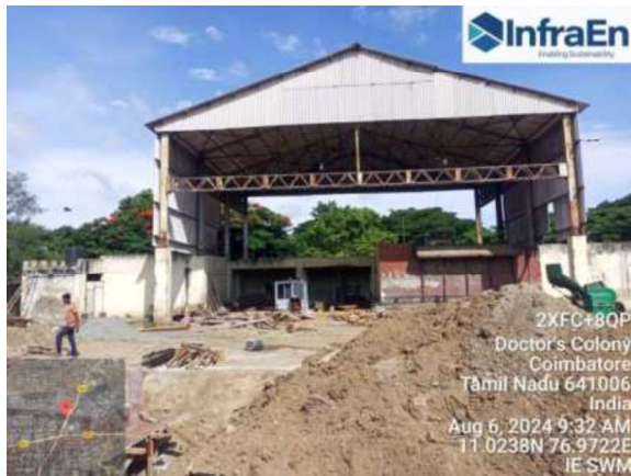
Sathy road transfer station construction work
